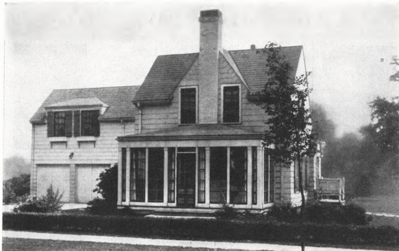
A two-story wing at the back, a sun porch, and other minor changes worked a transformation
